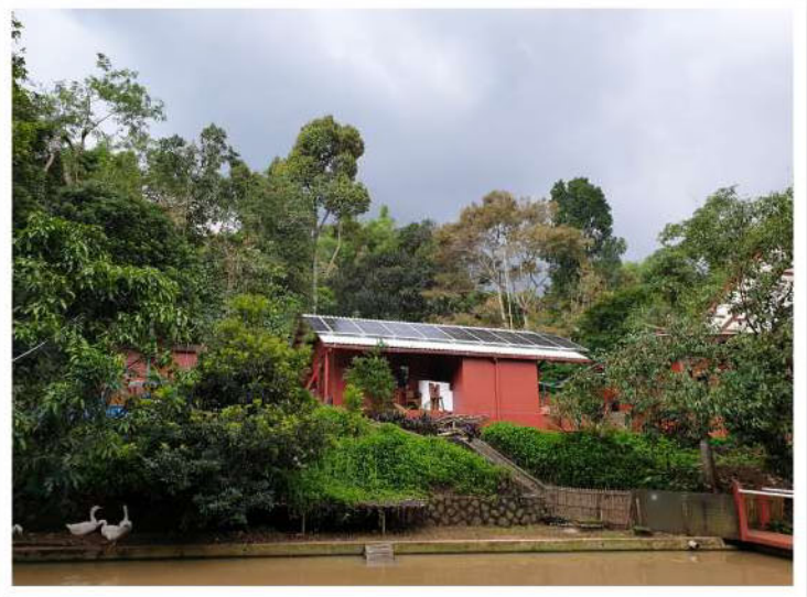
@ Bandung - 5 kW On Grid
